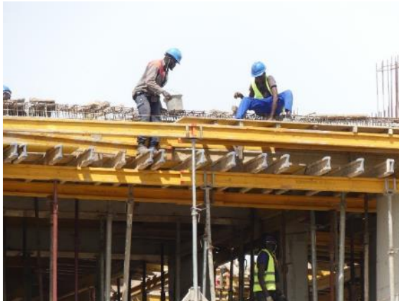
Building in progress
