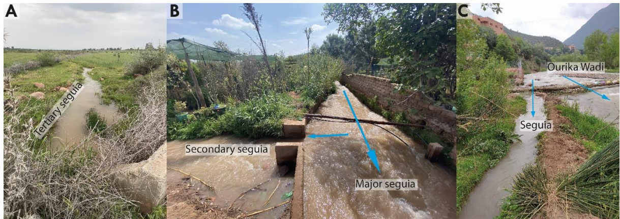
175 176 Figure 2: Photos of seguias from the study area, representing Seguias network in the piedmont; A: tertiary seguia irrigating 177 fields, B: secondary seguia uptake, and C: the major Seguia diverting water directly from the Ourika stream.
