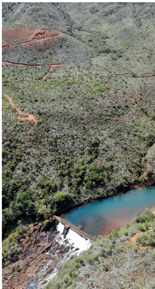
Barrage de Dumbéa – ©D. Gonzalez
