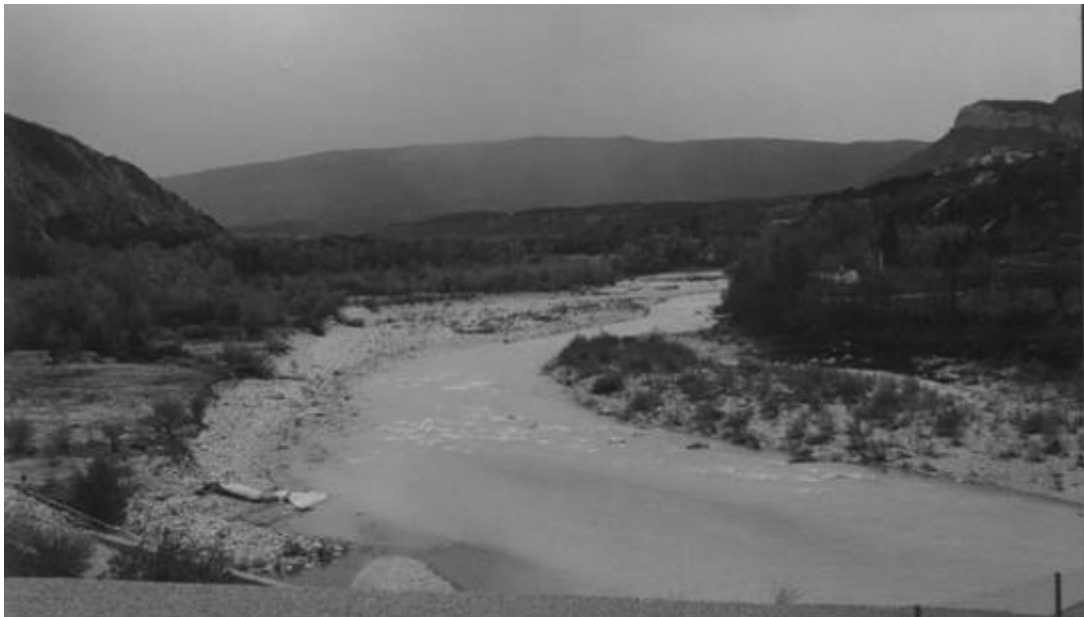
Fig. 5 The Buëch River valley immediately downstream from Saint Sauveur Dam (Hautes Alpes, France); the entrenchment of the bed (more than 3 m since 1992) in its own alluvium is detectable on both sides.
