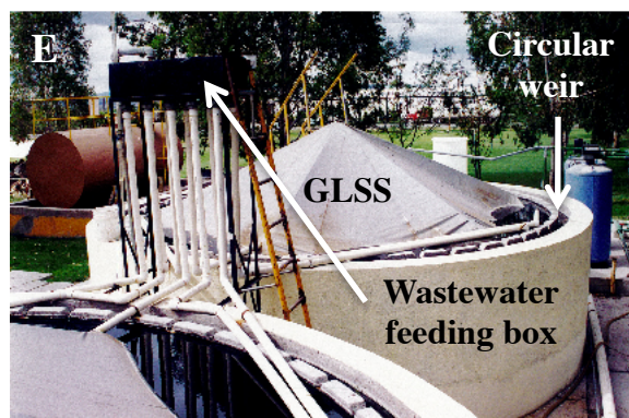
Figure 1. (A) Block process flow diagram of the cheese factory wastewater treatment plant, (B) general view of the plant with the homogenization tank in the front, the DAF system in the back right side and the two circular covered digesters before remodelling in the back left side, (C) view of the digesters before remodelling, (D) after remodelling, (E) detailed view of one of the digesters and of the wastewater feeding system (distribution box and pipes) after remodelling.
