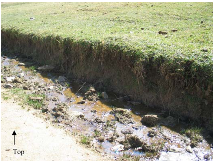
Fig. 14 Drainage pits in the wet grasslands
